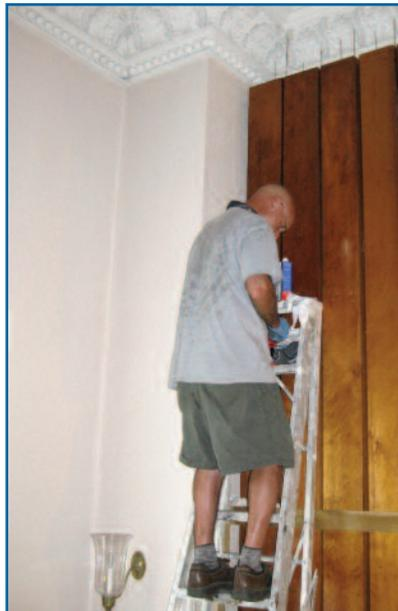
flank and form the exterior of the new instrument. These pipes were first restored with dowels and inserts replacing and cracks, languids checked and then, completely cosmetically stripped of old stains and shellac and three new coats of shellac applied during the summer. So the inside and outside of the instrument is now equally pristine and ready for the next century. It's worth a look up close if you care to venture up the balcony stairs.
